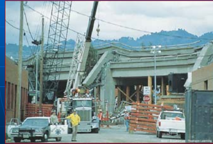
Damage in Oakland, CA, 1989
